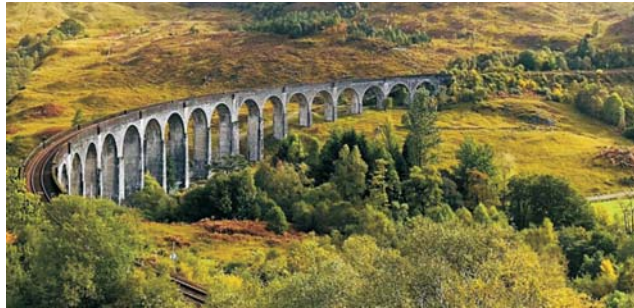
West Highland Railway
